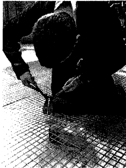
Apprentice cutting petal mesh
